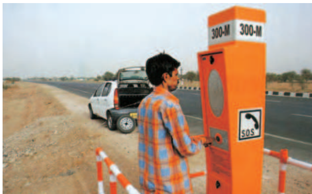
Fig. 7.10 : Emergency call box on NH-48
